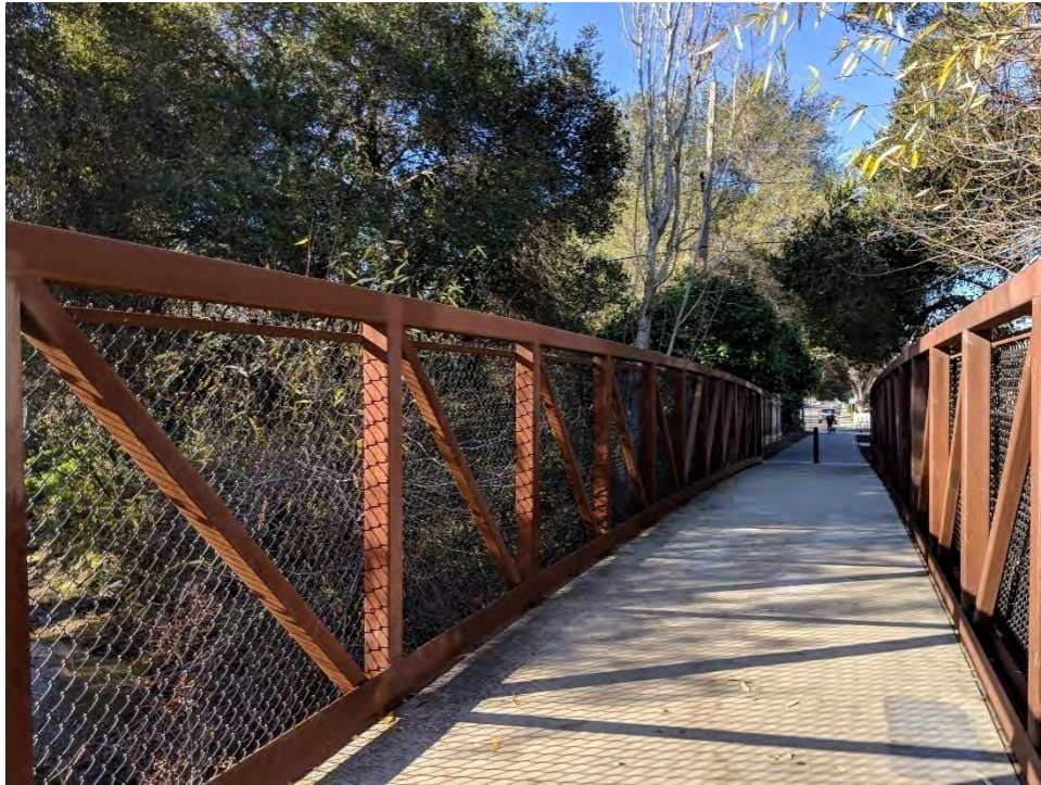
Pedestrian-bicycle bridge over Saratoga Creek. Picture looking west towards Sterling Barnhart Park.
