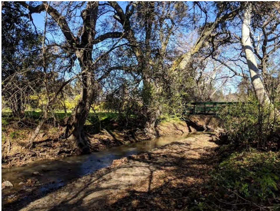
Pedestrian-bicycle bridge over Stevens Creek near Stockmeir Ranch. Picture looking north.
