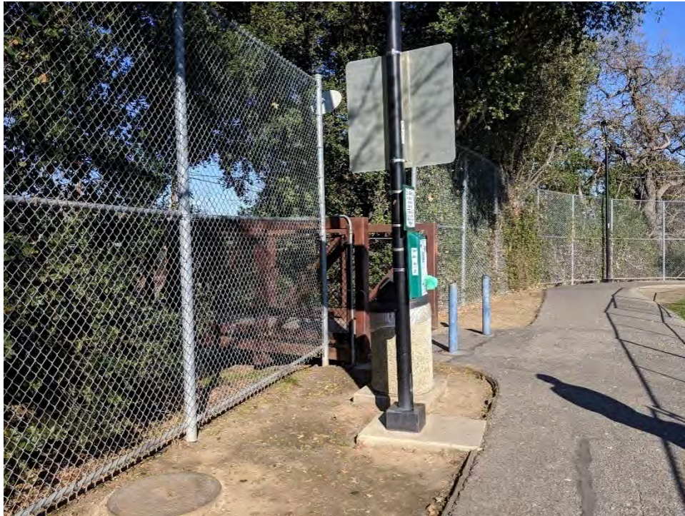
Pedestrian-bicycle bridge entrance to Creekside Trail. Picture from western edge of northern sport field in Creekside Park.
